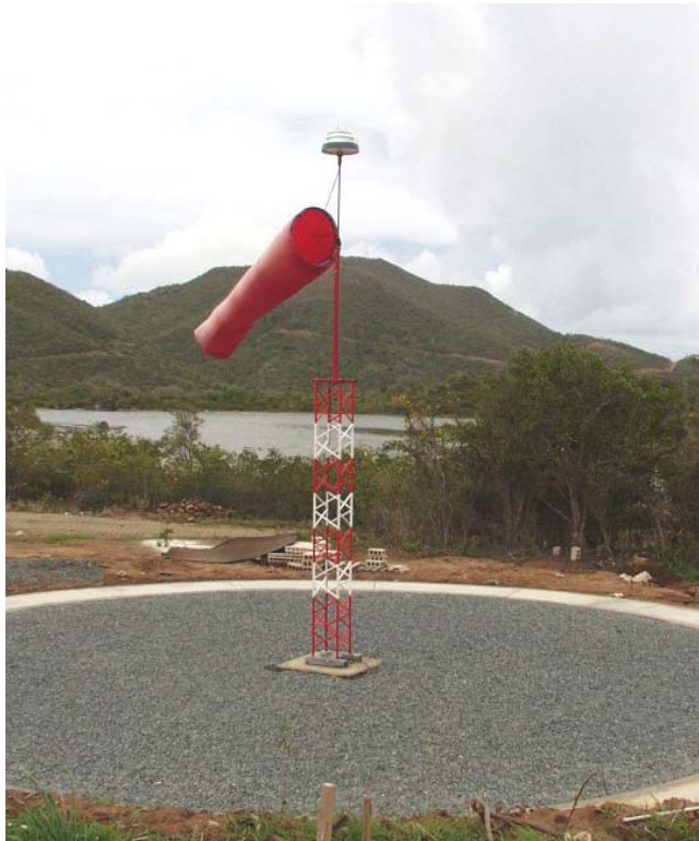
Externally illuminated wind cone
